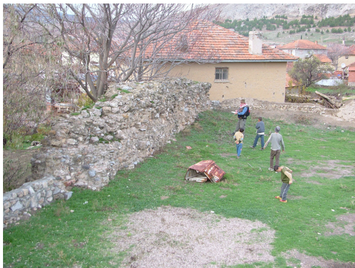
Fig 2. Inner face of the probable Roman fort wall at Işıklı showing its coursed rubble construction (photograph courtesy of B. Claasz Cockson).
