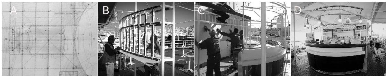
Figure 8a, b, c, d. Proposed orthogonal plan, Shelving unit frame building and final realization. Source: Siniša Prvanov.
