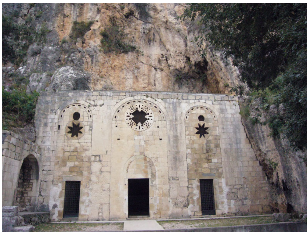
Fig. 1. The Cave Church of St Peter, one of the oldest churches in the world, is located at the outskirts of modern Antakya. (Copyright: Author)
