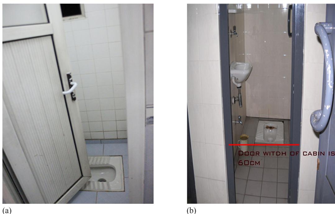
Figure 5. [In colour online.] Two examples of public toilets with inadequate access to stalls: (a) insufficient manoeuvring space; (b) narrow door.
