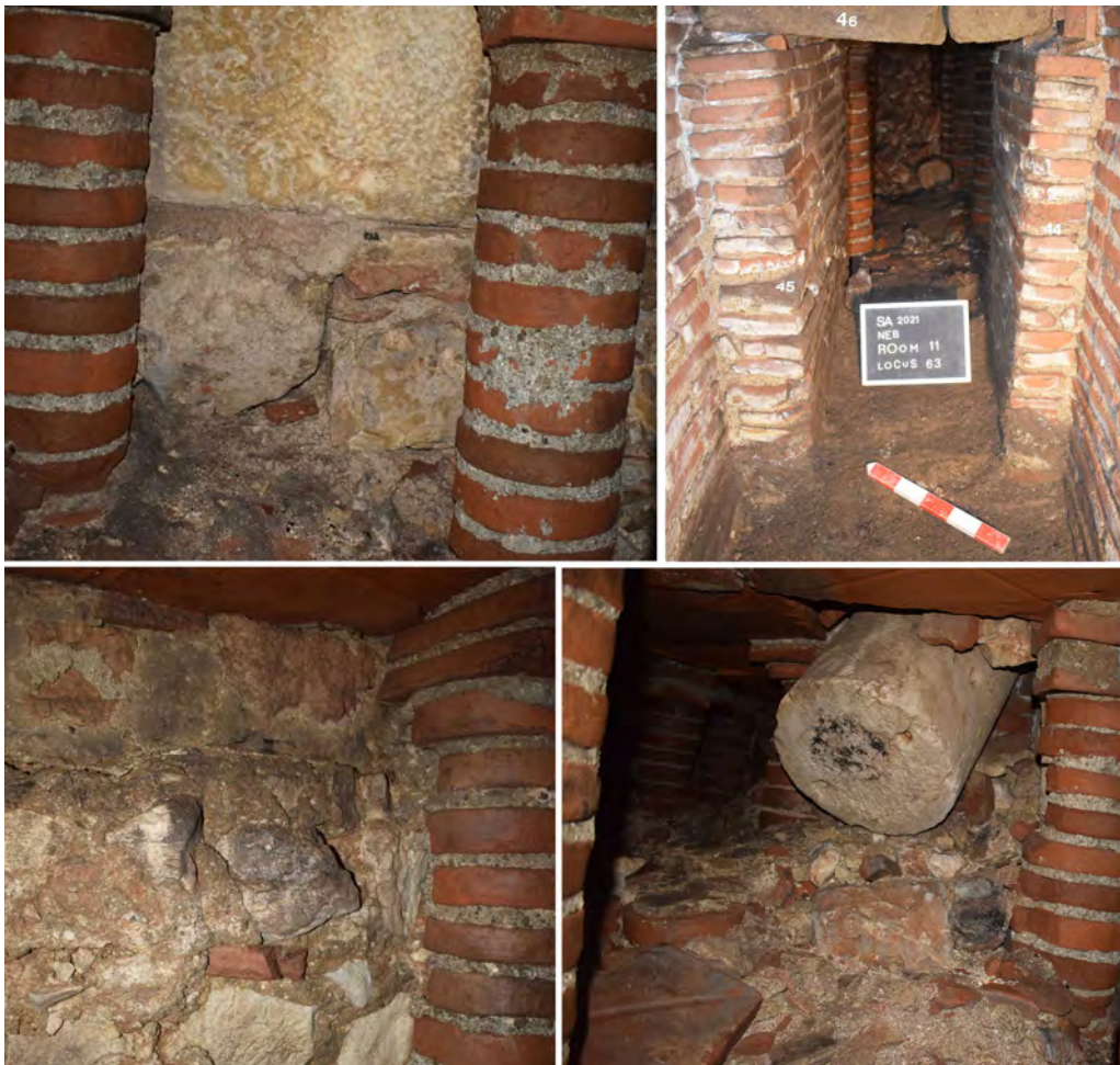
Fig. 29. (upper left) The mortared ashlar wall in the hypocaust of the northern wing. (upper right) The vaulted entrance and service corridor leading to the hypocaust. (lower left) The northern wall of the hypocaust. (lower right) The column which crashed through the ceiling of the hypocaust.
