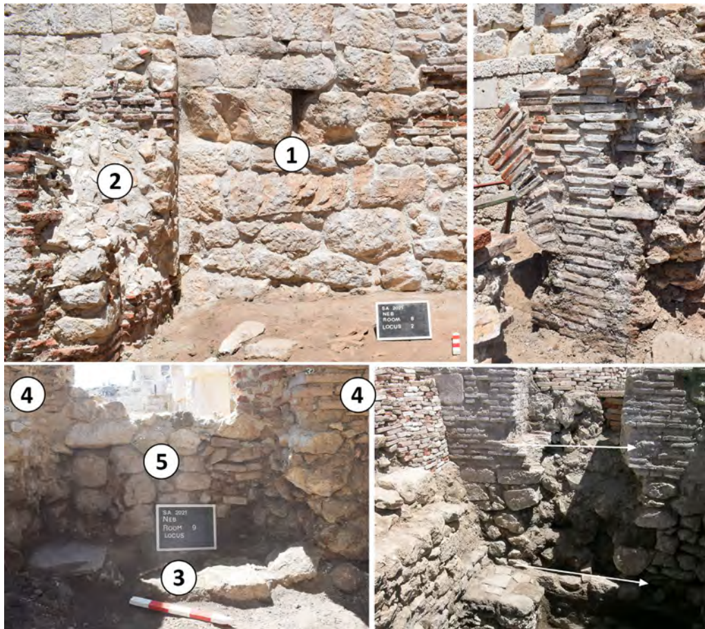
Fig. 50. (upper left) The (2) northernmost brick pier abuts (1) the 350/400-450 CE inner face of the northern wall. (upper right) The spring in the brick pier connecting to the WE oriented arcade. (lower left) Eastern view of the northernmost entrance in between two piers, including (3) the threshold, (4) the brick piers, and (5) a 550-650/75 CE blockage wall. (lower right) Western view of the southernmost entrance in between two piers, including the 350/400-450 CE threshold (upper arrow), and the 550-650/75 CE threshold aligning with the later floor (lower arrow).
