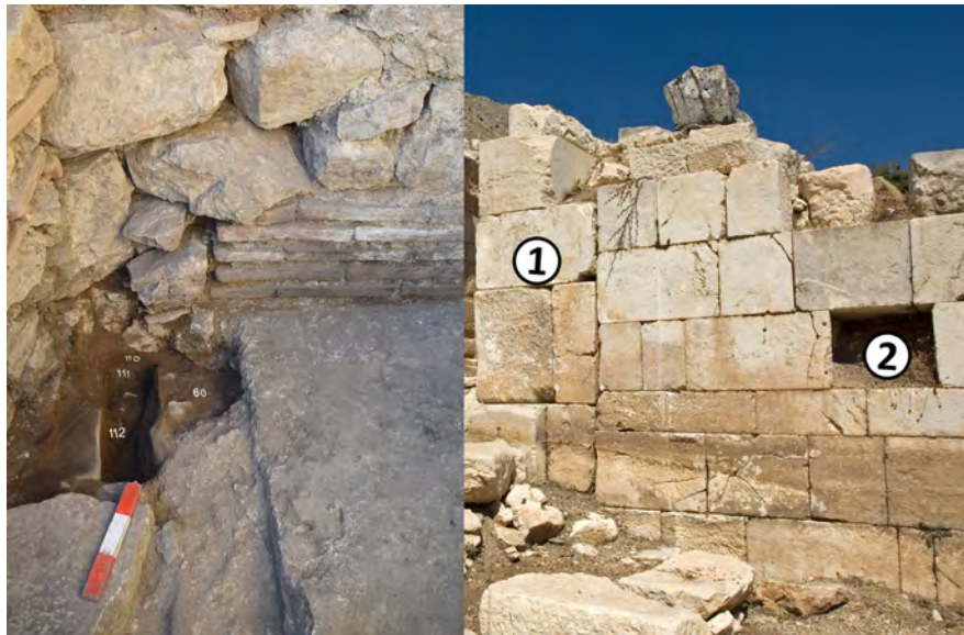
Fig. 46. (left) The profile where the easternmost part of the northern wall's inner face was placed on the WE oriented segment of the 75-125 CE wall. (right) The north-western corner of the late antique Agora Building, where (1) the double northern wall and (2) northwestern wall connect. © Sagalassos Archaeological Research Project .
