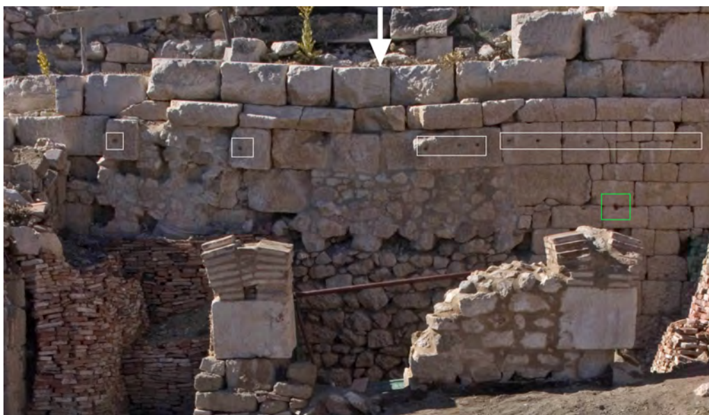
Fig. 44. Southern view of the western segment of the northern wall. Indicated are the area where the wall sags (arrow), the continuous line of clamp holes (white rectangles), and the clamp carved in between two blocks (green rectangle). © Sagalassos Archaeological Research Project .
