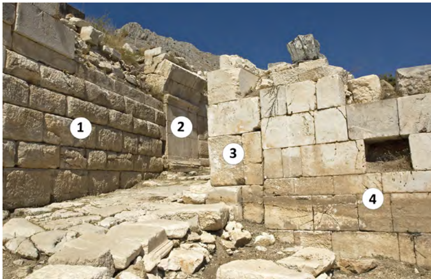
Fig. 3. SW view of the NE corner of the Upper Agora. Indicated are (1) the 150-100 BCE Terrace Building, (2) the 1-50 CE Northeast Gate, (3) the 350-400/450 CE northern wall of the late antique Agora Building, and (4) the western ashlar segment. © Sagalassos Archaeological Research Project.
